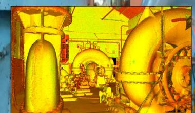
The powerhouse was built in 1923 by Logan City and is located about two miles up Logan Canyon. McNeil Engineering used 3D Laser Scanning technology (LiDAR Scanning) on this project to create a highly accurate representation of the existing conditions of the powerhouse to aid in the design and installation of new mechanical equipment and future modifications.
